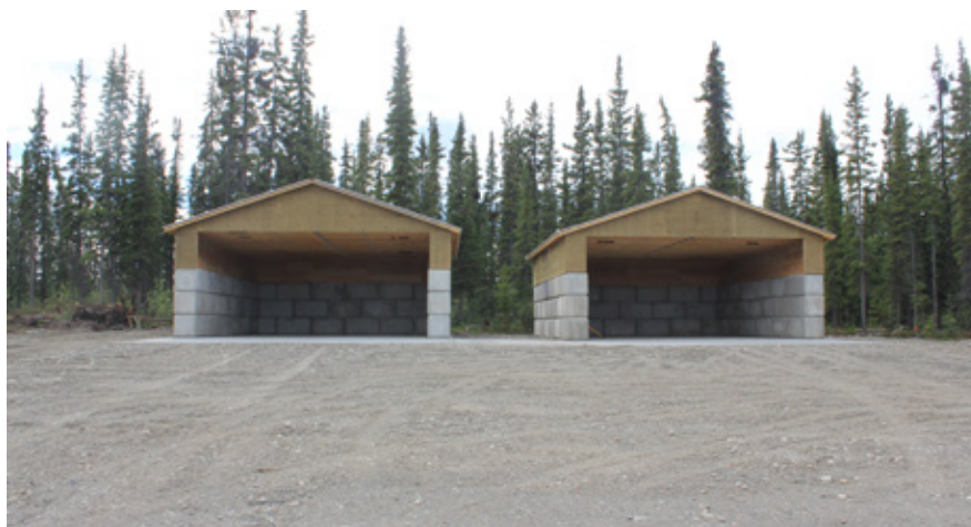
Biomass storage building for the wood chips
